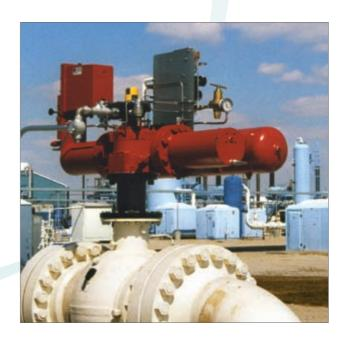
The gas control manifold employs poppet style control valves – a reliable design trusted throughout the industry. They are pilot operated for remote control. Operation is simple and intuitive.
